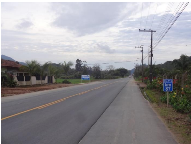
Recapeamento executado - km 87,0
